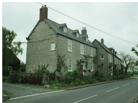
Above: Masons Farm in Oxfordshire
