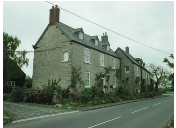
Above: Masons Farm in Oxfordshire
