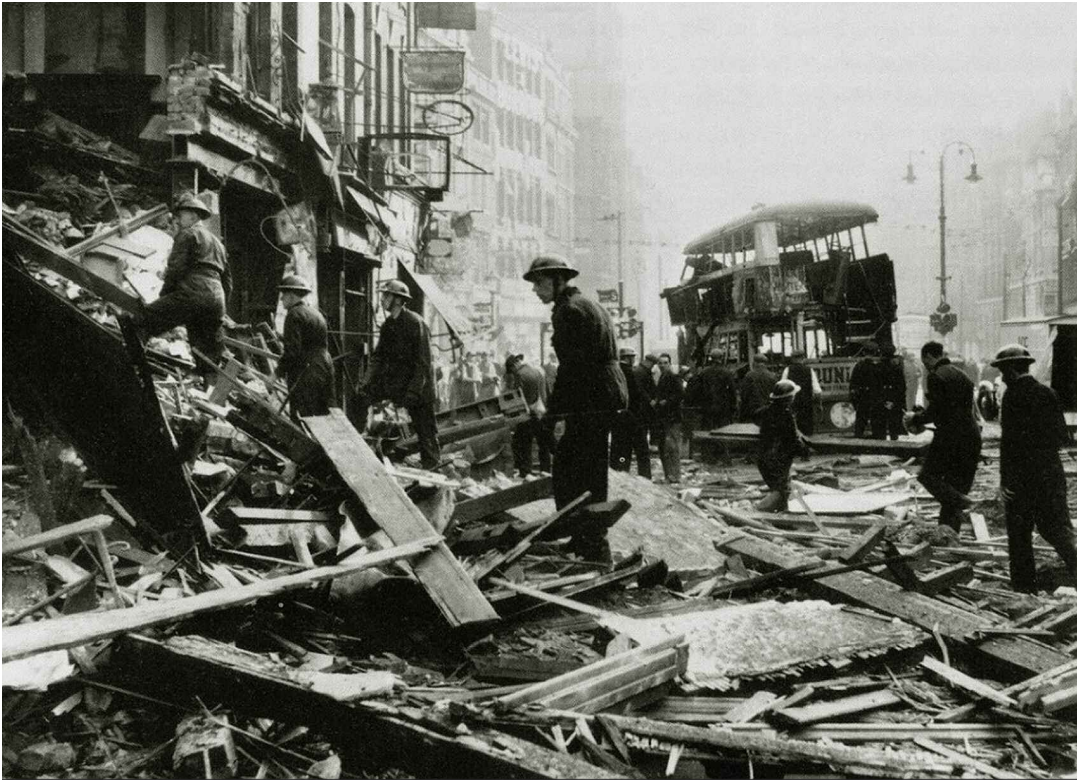
Above: A scene of devastation as rescue workers attend to bombed buildings outside Chancery Lane station on High Holborn, close to the junction with Gray's Inn Road, looking east, on Tuesday 8 October 1940. The German bombers attacked the area at around 9am during the morning rush hour, killing 32 people.
